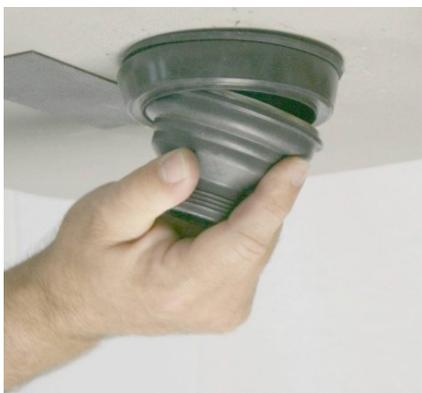
Insert drain lip into seal
