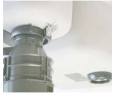
Support disposer with one hand and attach clamp.
