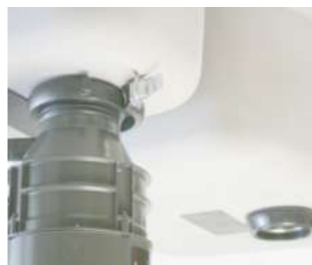
4. Support disposer with one hand and attach clamp.
