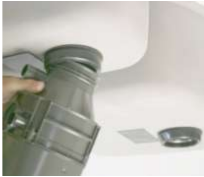
Slip the lip into the the rubber mount.
